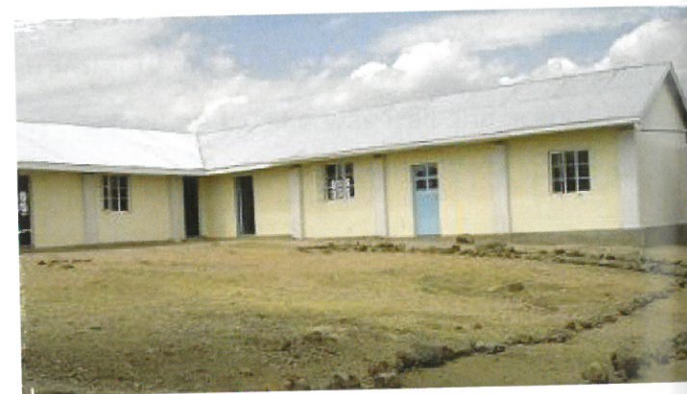
Kopala Primary school after renovation
