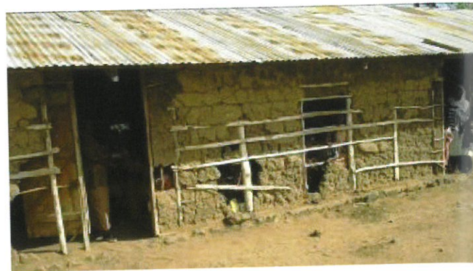
Aringo Primary school before renovation
